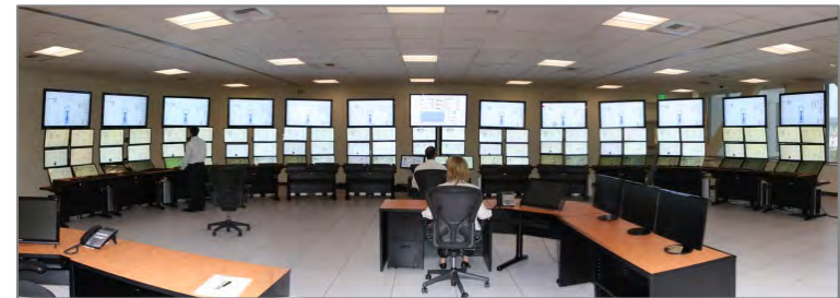
NuScale Control Room Simulator
