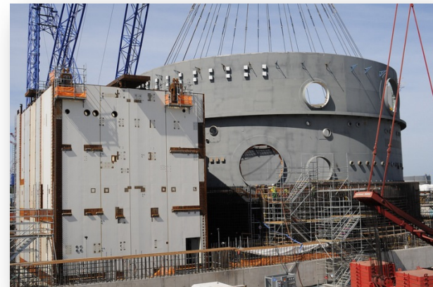
SCE&G Places First Ring on V.C. Summer Unit 2 Containment Vessel, June 2014 ©SCE&G
