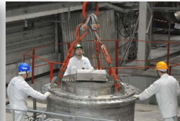
Refuel floor during the recent first-time fueling of BN-800 (Rosatom)
