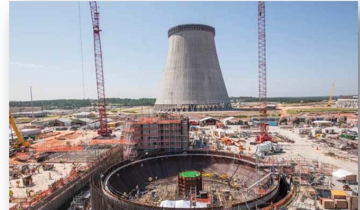
Construction of Vogtle Unit 3, August 2014 ©Georgia Power Company
