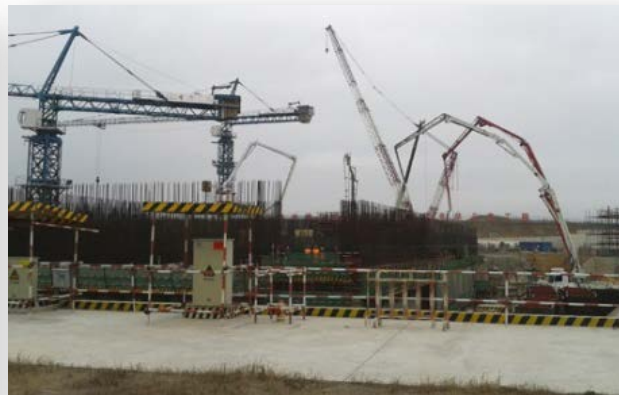
The construction site of the first HTR-PM at Shidaowan (Image: CNEC)
